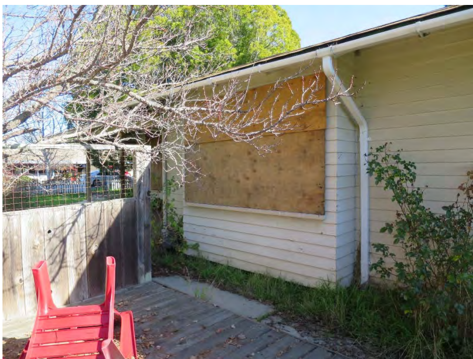
Figure 16. Shallow pop-out on the west facade, view northeast (ARG, January 2019)
