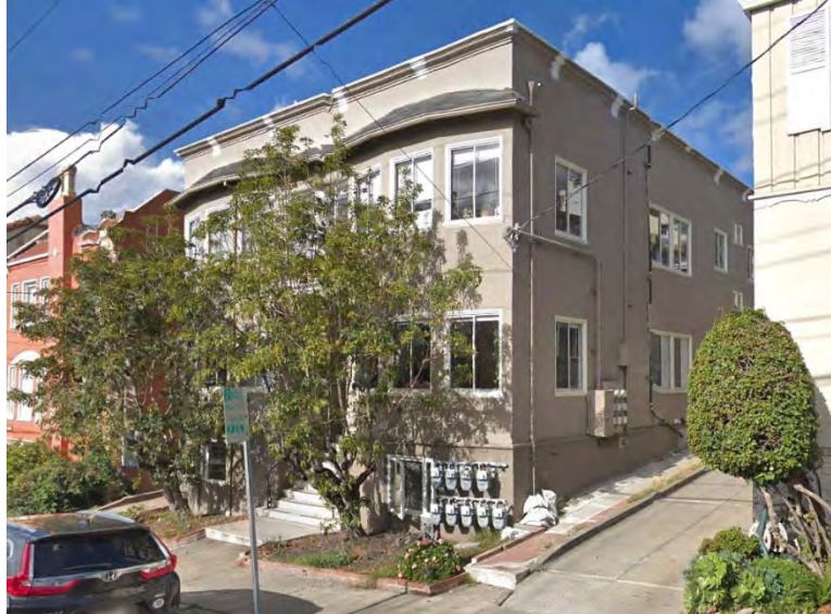
Figure 9. 2517 Virginia Street, Berkeley (Google Earth)
