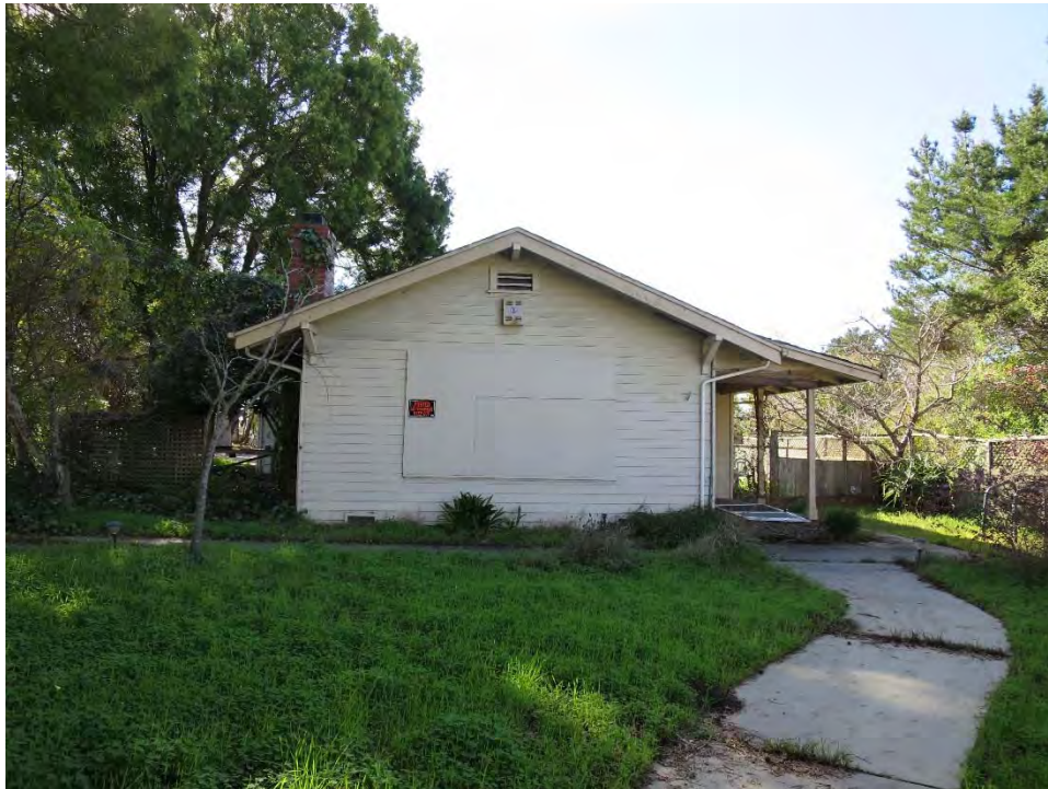
Figure 14. North façade, view south (ARG, January 2019)
