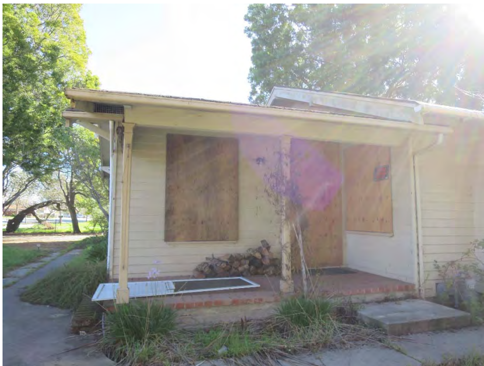
Figure 15. Porch on the west façade, view east (ARG, January 2019)
