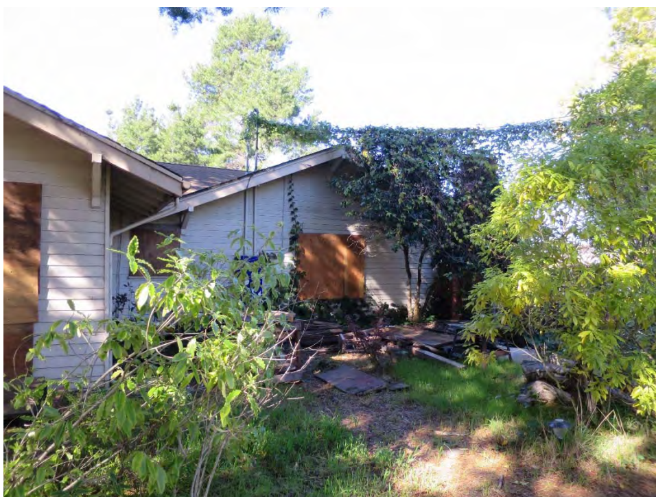
Figure 20. East façade, view west (ARG, January 2019)
