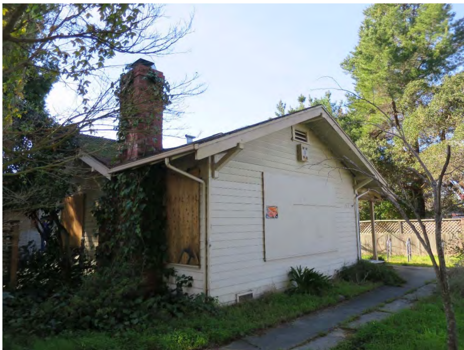
Figure 21. Exterior brick chimney on the east façade, view southwest (ARG, January 2019)
