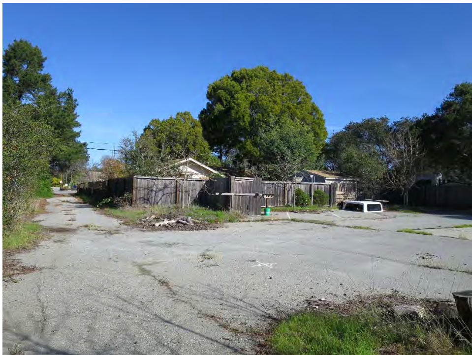
Figure 26. Rear paved area, view northeast (ARG, January 2019)
