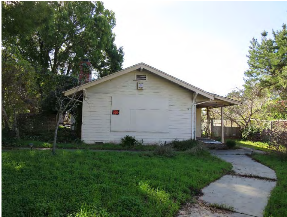
Figure 14. North façade, view south (ARG, January 2019)
